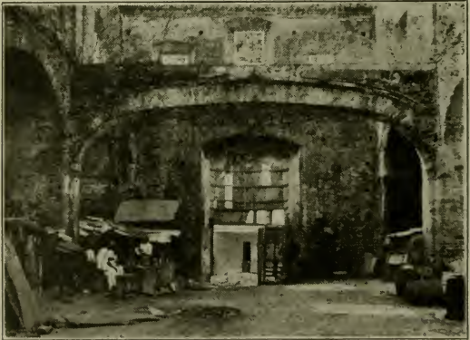
FLAT ARCH IN CHURCH OF SANTO DOMINGO—PANAMA.
